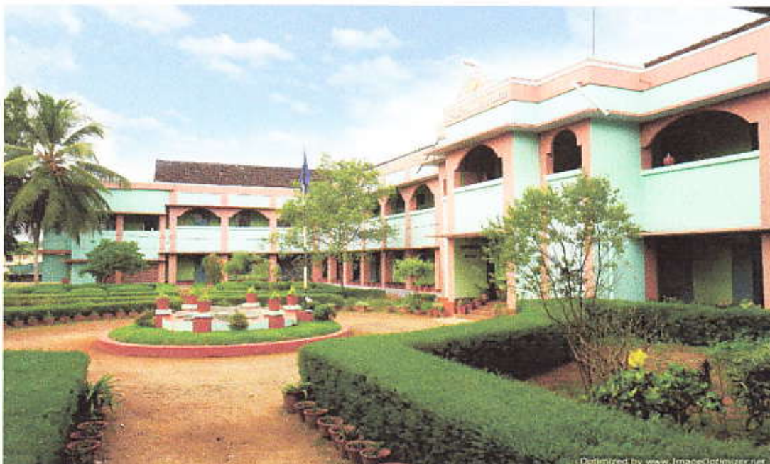
Rear view of the building
